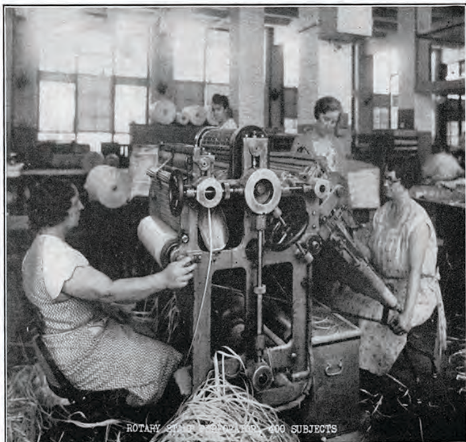
Fig. 2—MANUALLY OPERATED PERFORATING MACHINE.
