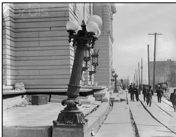
A photograph showing the buckling of the pavement and bent lamp post in front of the Post Office.
